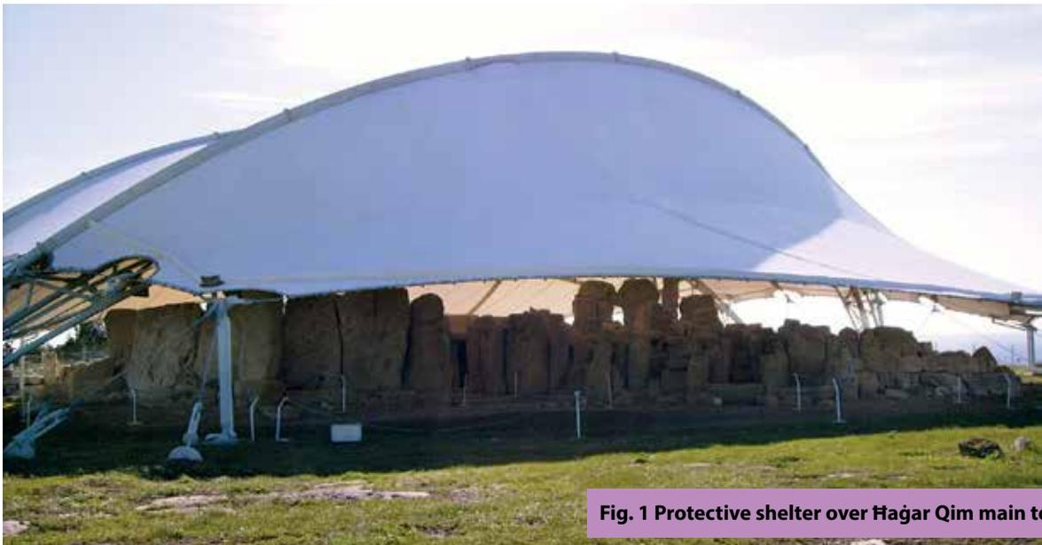
Fig. 1 Protective shelter over Ħaġar Qim main temples
