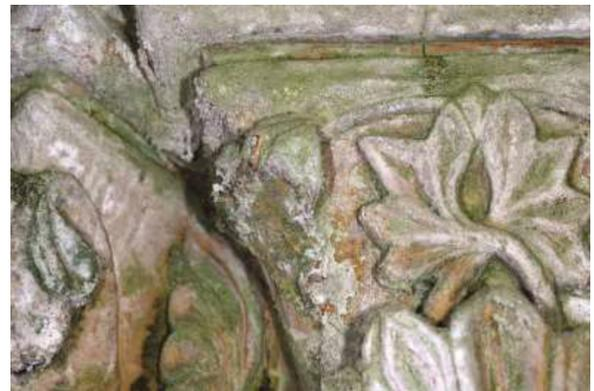
**Fig. 3.** Algae, bacteria and cyanobacteria are pioneer microorganisms which can cause significant colour alterations on stone, as displayed by the green and white shades seen above.
