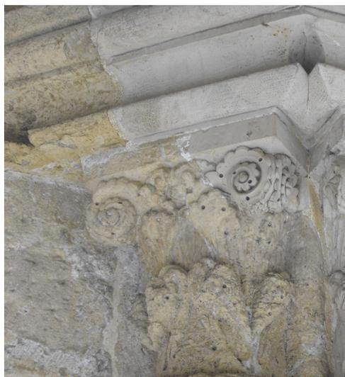
Fig. 1. Two types of limestone (yellow and white) were used for the construction and punctual rehabilitation of the Old Cathedral in Coimbra.
