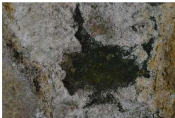
Fig. 4. Algae growing on a stone substrate where water is readily available. They form powdery or viscous layers and, as seen here, are responsible for dramatic chromatic changes.
