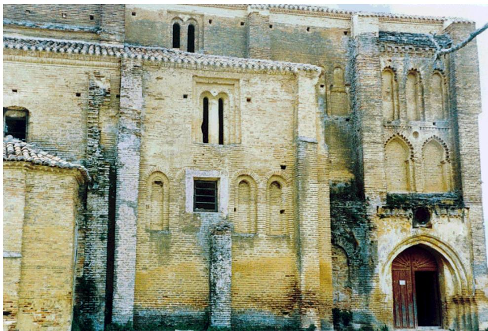
**Figure 1.** Convento de la Peregrina, Sahagún, León, Spain. The extensive white coverage of the outer walls to the left of the entrance door due to colonies of *Diploschistes scruposus* is significant. The unglazed window apertures should also be noted.
